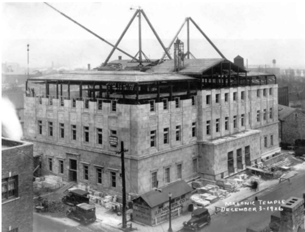
Figure 8. Construction progresses, December 1926.
