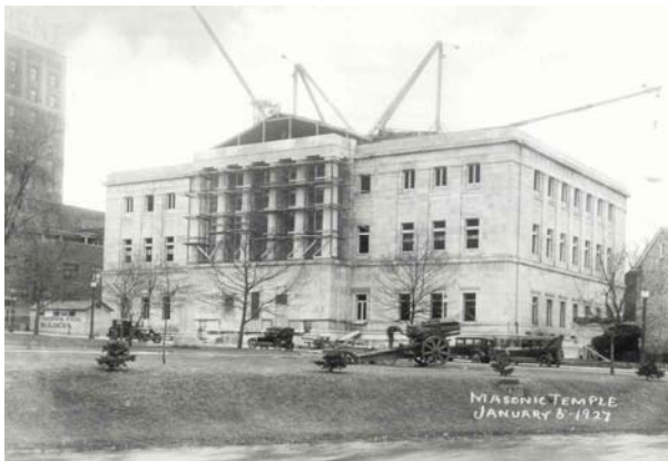
Figure 9. Exterior construction nears completion, January 1927.
